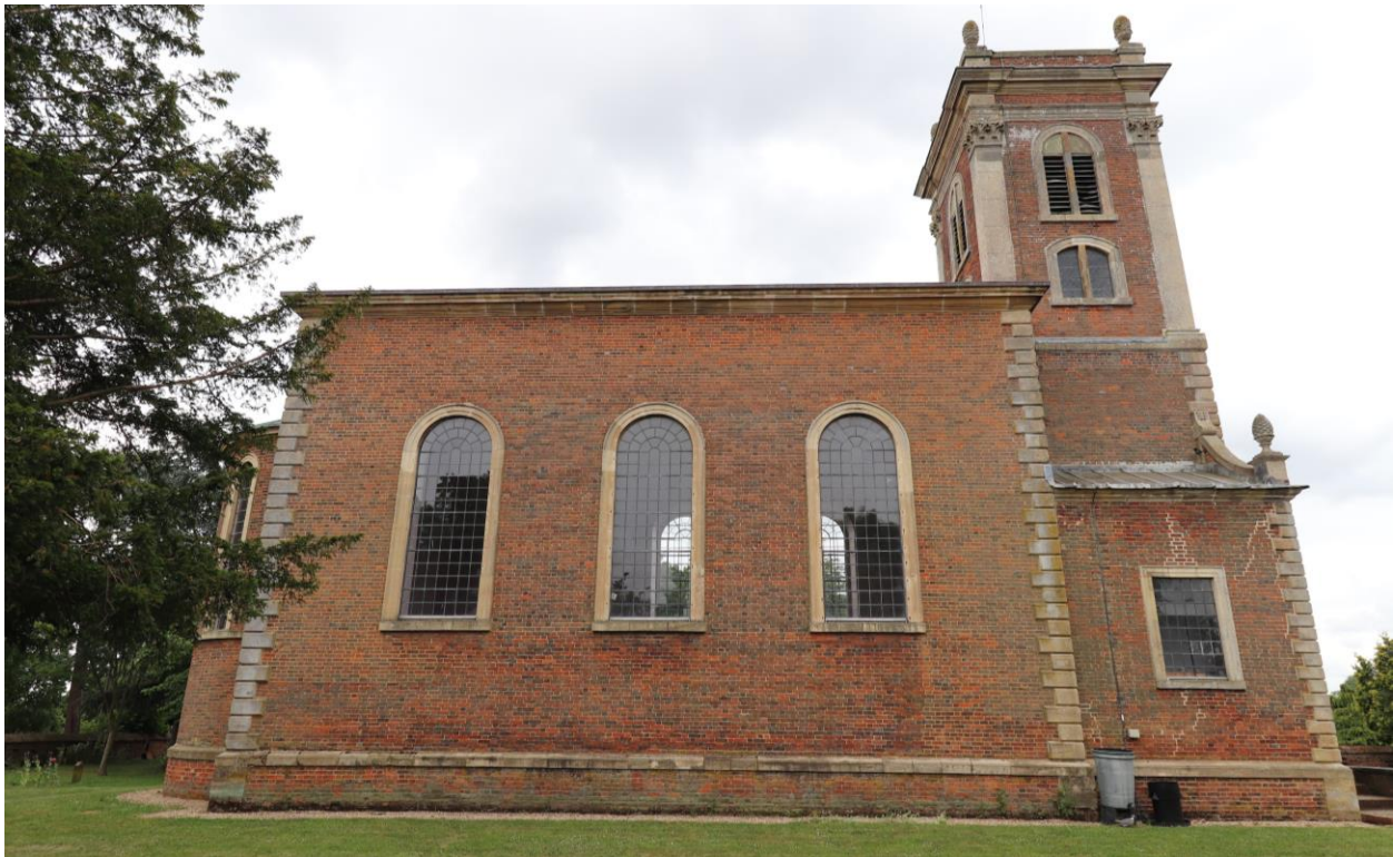
Above: North elevation of the church
