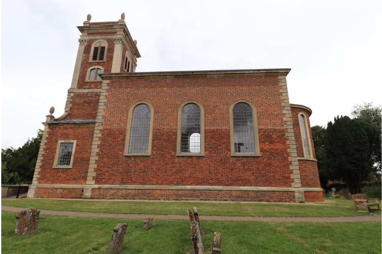
Above: South elevation of the church. Note the jarring effect at high level on the nave wall, the result of a different pointing style
